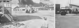
9:11 a.m. Main support of building gives way as steel cable is hauled in by powerful winch attached to bulldozer in tight back-ground. 9:15 a.m. Sopotencion mayor di e edificio ta laga basha mientras e cable di staal ta wordo hala door pa medio di un potente winch masá adiantu di un bulldozer atras hasda drecha.
